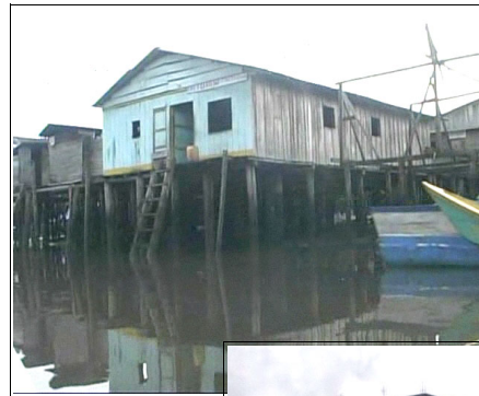
House made of wood, builded over stakes
