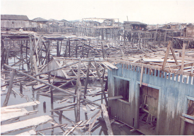
Picture 7. Destruction of pile-supported housings, Tumaco 1979.
